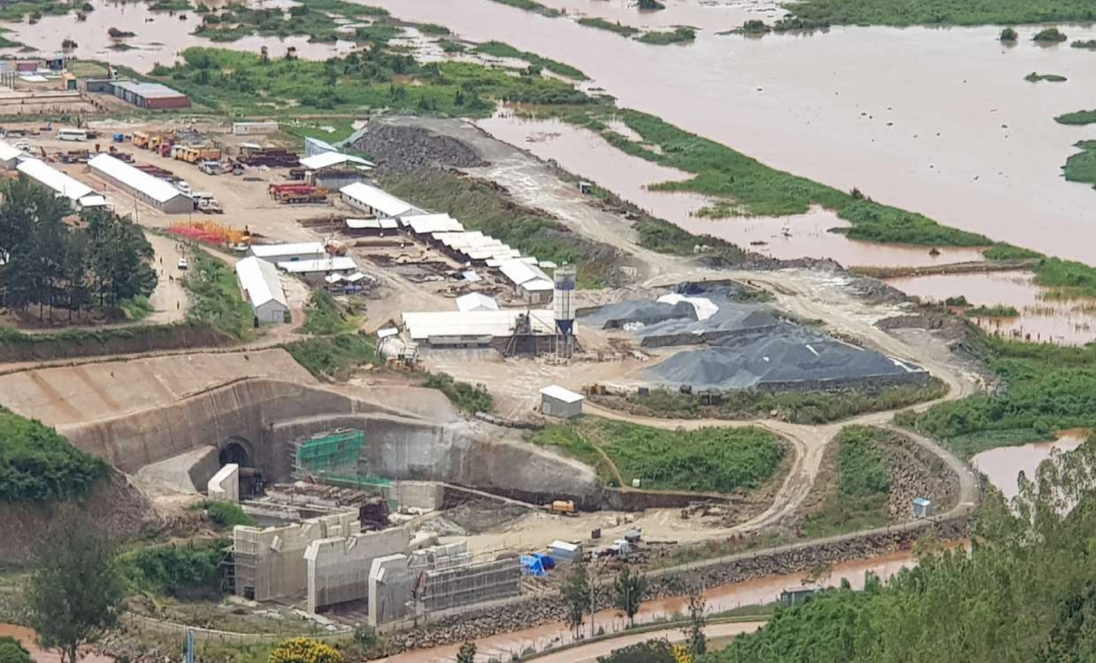
ONGOING CONSTRUCTION AT THE REGIONAL RUSUMO FALLS HYDROELECTRIC PROJECT
