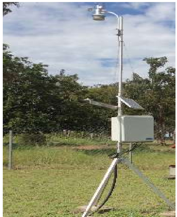
AN AUTOMATIC WEATHER STATION INSTALLED BY NELSAP
