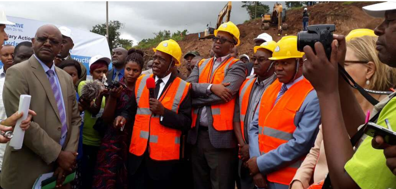
HON. PROF. SOSPETER MUHONGO THE MINISTER OF ENERGY-TANZANIA, HON. COME MANIRAKIZA, THE MINISTER OF ENERGY-BURUNDI AND HON. JAMES MUSONI THE MINISTER OF INFRASTRUCTURE-RWANDA, MEET THE PRESS AFTER RUSUMO FALLS HYDROELECTRIC PROJECT CONSTRUCTION LAUNCH
