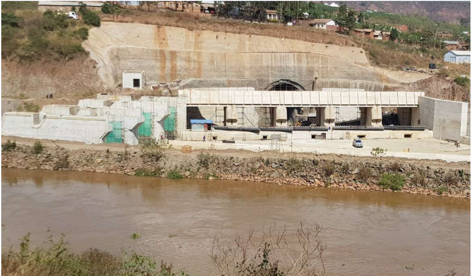
ONGOING CONSTRUCTION AT THE REGIONAL RUSUMO FALLS HYDROELECTRIC PROJECT (RRFHP) SITE
