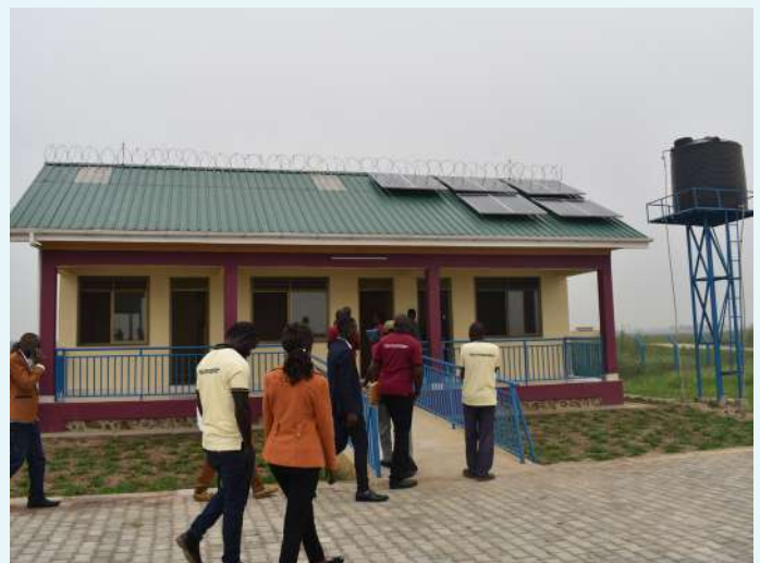
FISHERIES OFFICER'S OFFICE AND ADMINISTRATION BLOCK AT RWENSHAMA LANDING SITE IN UGANDA
