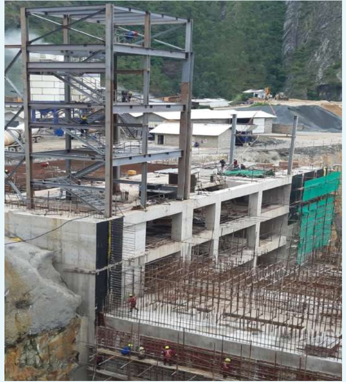
SERVICE BAY AT THE POWERHOUSE
