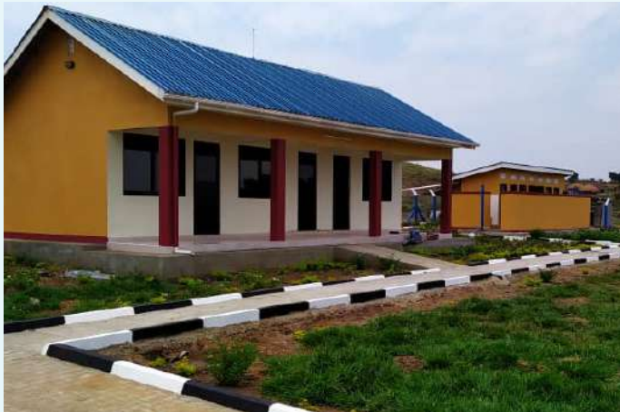
ADMINISTRATION BLOCK AND 'ECOSAN' SANITATION SECTION OF MBEGU LANDING SITE ON LAKE ALBERT, UGANDA
