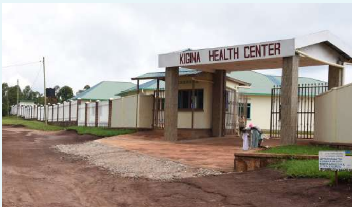
KIGINA HEALTH CENTRE BUILT THROUGH THE LADP PROGRAM OF RUSUMO PROJECT, SERVES 10,000 PEOPLE
