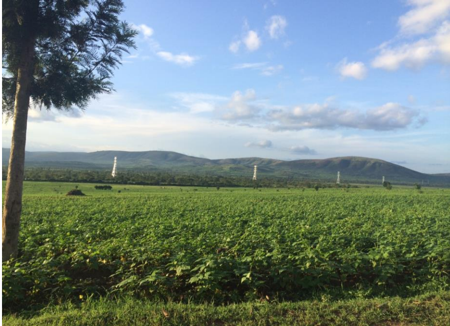
Rwanda to Uganda Interconnection (Mirama-Shango)
