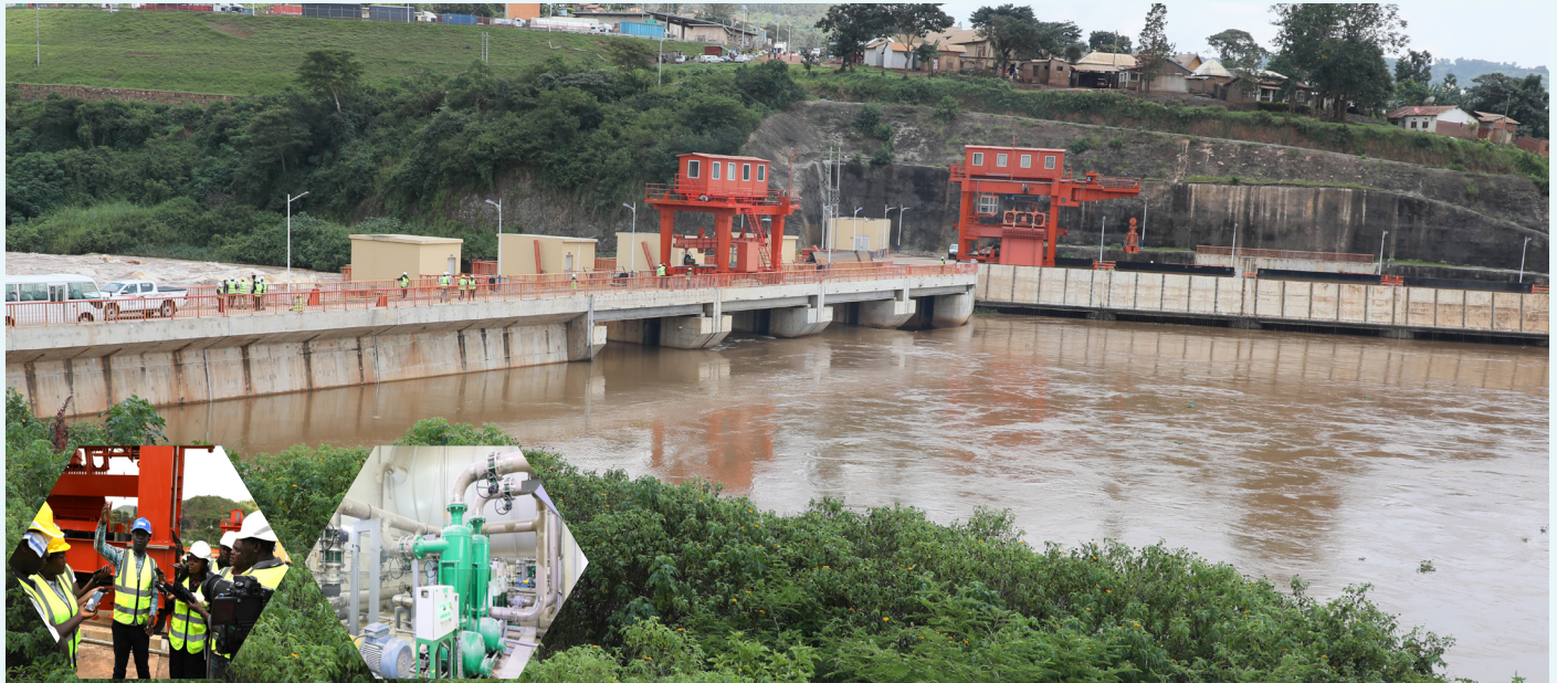
A SECTION OF THE POWER HOUSE AND COMPLETED POWER INTAKE SECTION OF THE RUSUMO PROJECT SHOWING THE RADIAL GATES AND HEAD RACE TUNNEL (PARTLY OBSCURED) INSET 01: THE RUSUMO PROJECT MANAGER ADDRESSING JOURNALISTS FROM SEVEN NILE EQUATORIAL LAKES COUNTRIES WHO HAD VISITED THE PLANT ON 31ST JANUARY 2024. INSET 02: A SECTION OF THE POWERHOUSE
